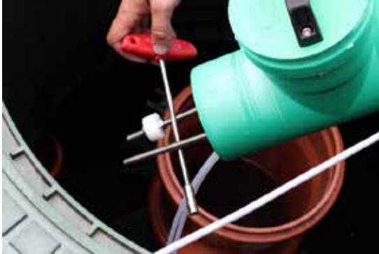
Figure 27: Performing a function test of the electrodes.
