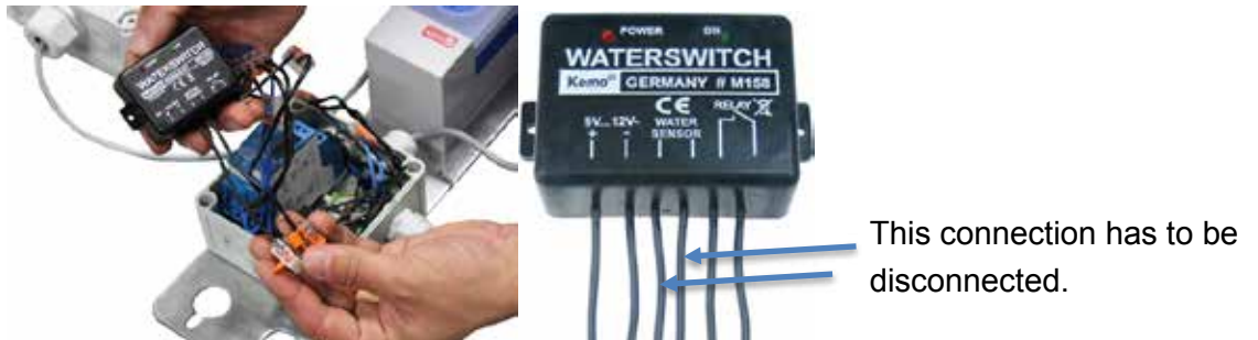
Figure 18: Disconnection of the electrical wires which are connected to the watersensor.
