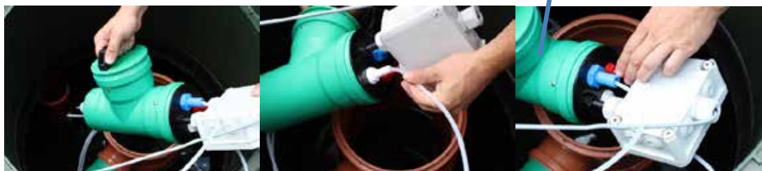
Figure 13: Installation of the 6 mm chlorine dosing hoses in a chlorine tank (e.g.: Saphir tank).
