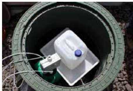
Figure 8: Mount the drip pan onto the plug connection in order to store the bleach solution inside the chlorine tank.
