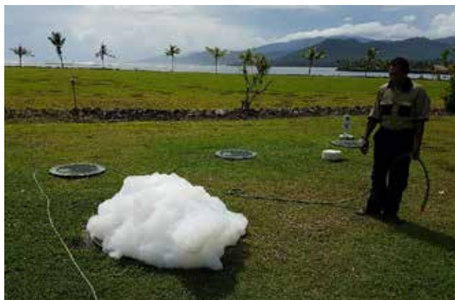
Extreme foam formation while cover is open
