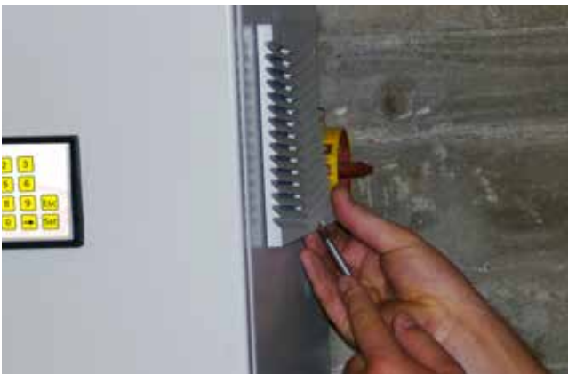
Removal of the ventilation screen
